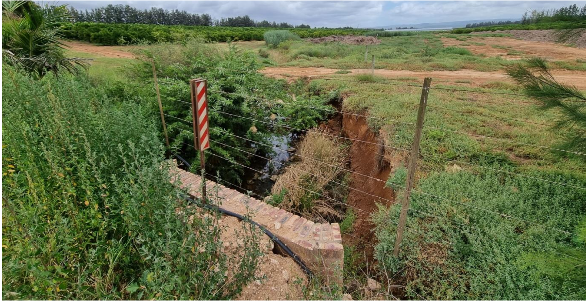
Figure 7-6: Instream road bridge and culvert to allow water pass-through at CDDS2 with bank erosion (September 2021)
