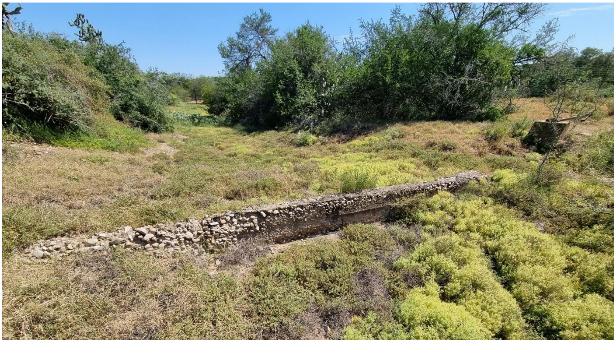
Figure 7-5: Small scale deteriorated instream weir across the channel at CTUS (January 2022)
